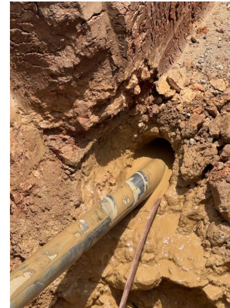
Installing the conducting electrode using HDD
