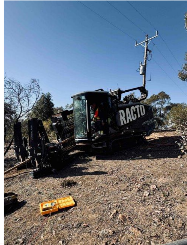
Trenchless Grounding Work Site in Australia
