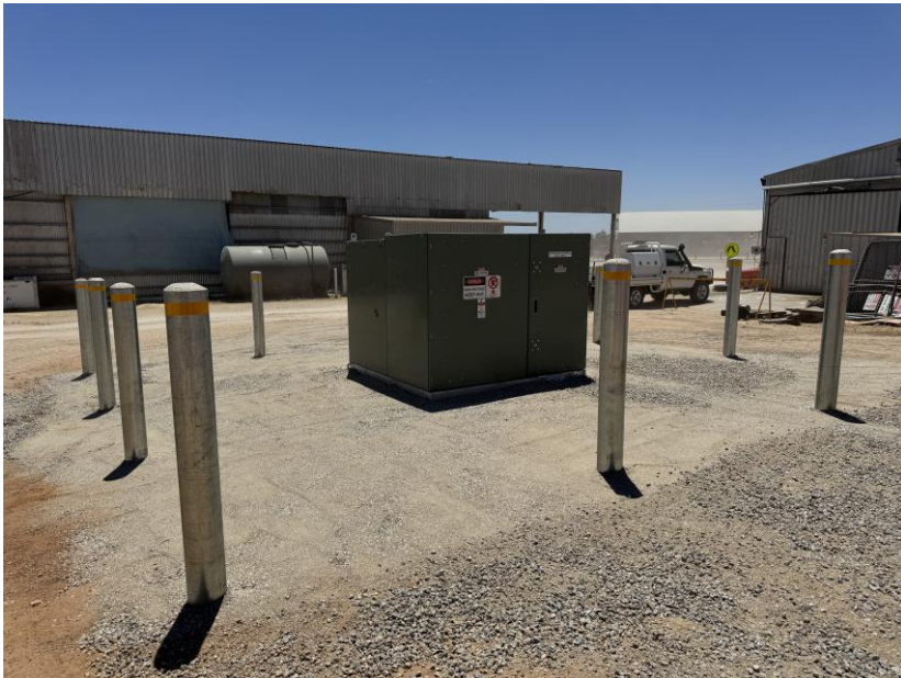
Ground Mounted HV / LV Transformer Replacement
