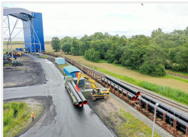
Shortly before completion: In mid-December, OGE connected the WAL pipeline to the German natural gas network via the North German Natural Gas Transversal (NETRA) pipeline. © OGE
