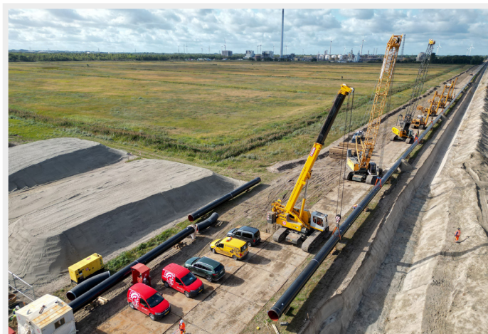
Pipeline being lowered into the trench © OGE
