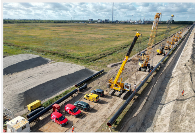
Pipeline being lowered into the trench © OGE
