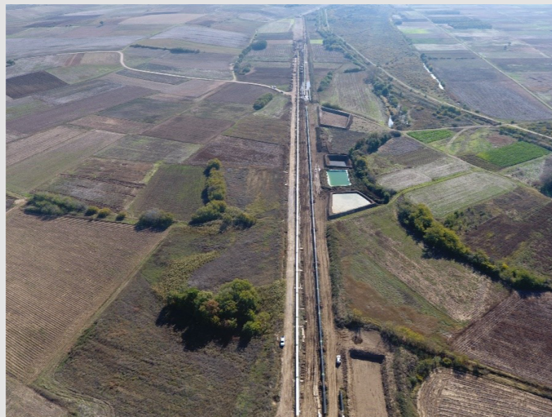
Figure: Overview of the Pipe Site
