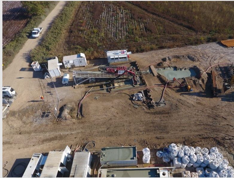
Figure: Overview of the Rig Site
