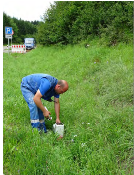
Fig. 8: Detection of the drill head along biologically valuable roadside
