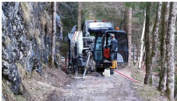
Fig. 1: Drilling under a narrow mountain-path
