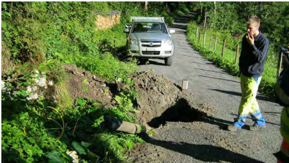
Arrival of the drillhead in the target pit
