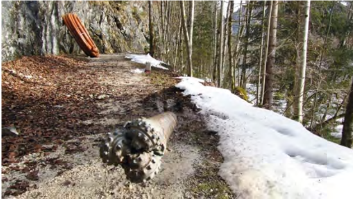
Fig. 2: The Rockbreaker drillhead arrives at the target-side
