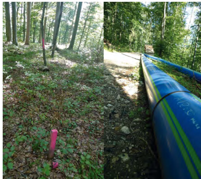
Fig. 14: Drill-path with markings and pipe layout
