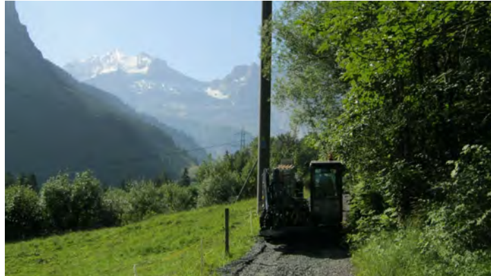
Fig. 4: Grundodrill 18ACS on its way to the job site in self-drive-mode
