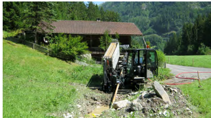
Fig. 5: Drill rig at the starting pit, boulders directly underneath the surface
