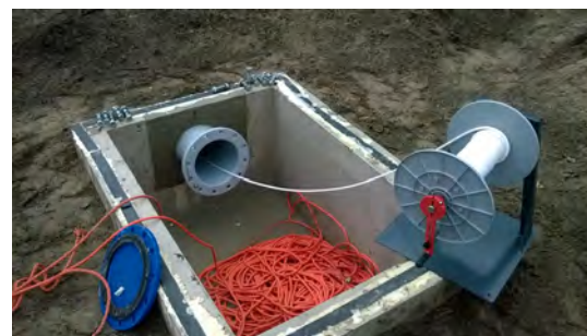
Fig. 11: HDDW just after installation
