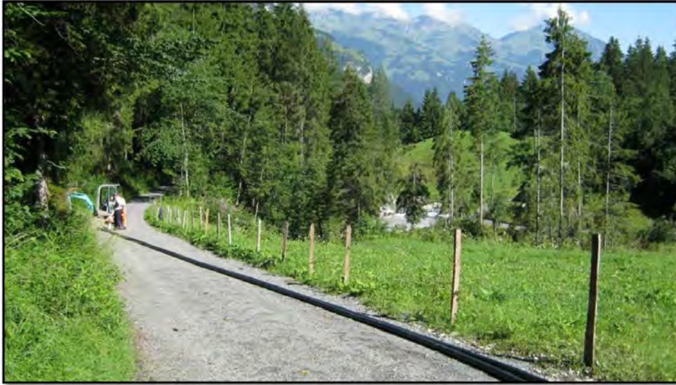
Last step: Pulling the pipes into the drill hole
