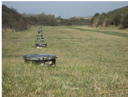
Fig. 4: Many vertical wells need to be installed to reach the required capacity in a thin aquifer
