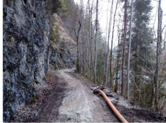
Fig. 3: Pulling in the sewer pressure pipe
