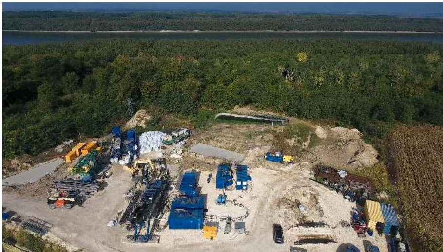
Picture 02: Jobsite HDD1 View from East to West
