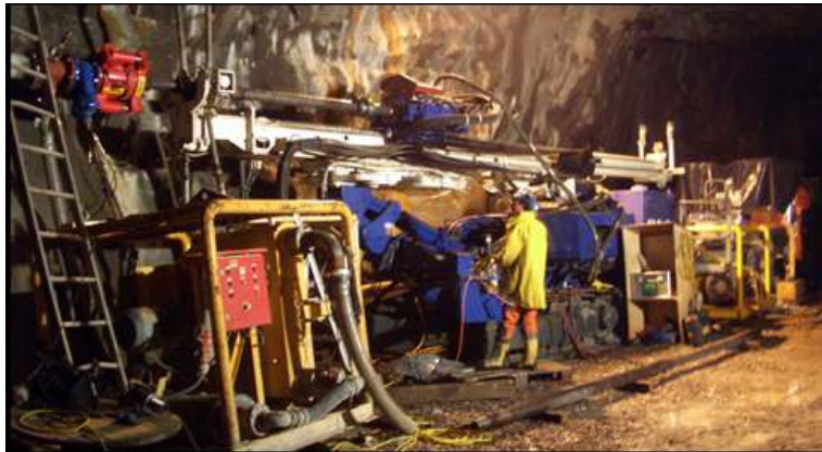
Rig used on Freeze hole drilling in Hallandsas
