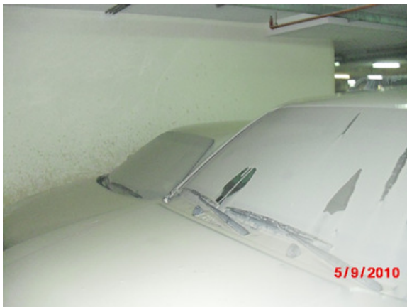
Cars in underground carpark covered in bentonite
