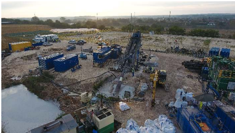
Picture 03: Jobsite HDD1 View from West to East
