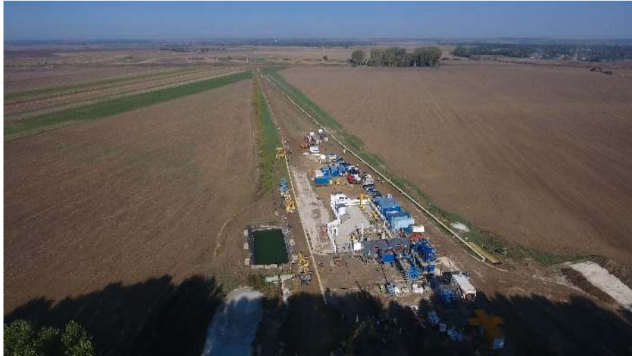
Picture 01: Pipe Trace
