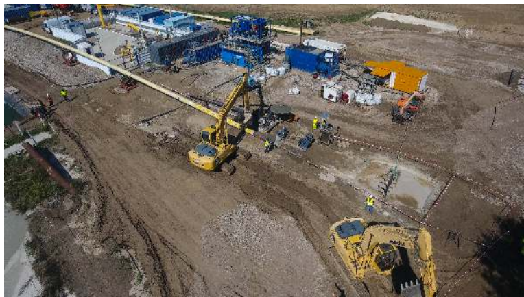
Picture 05: Exit point pull back HDD1
