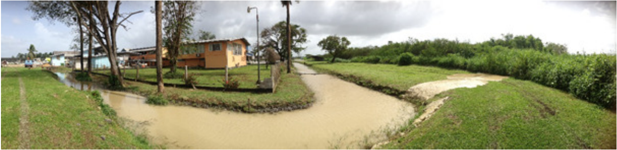
Frac out of mud into a ditch in Suriname
