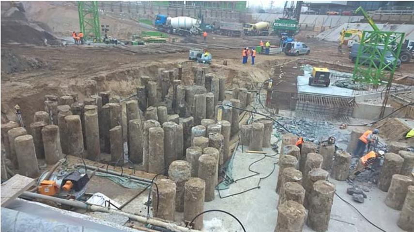
Figure 8: parts of the foundation required very dense pile groups
