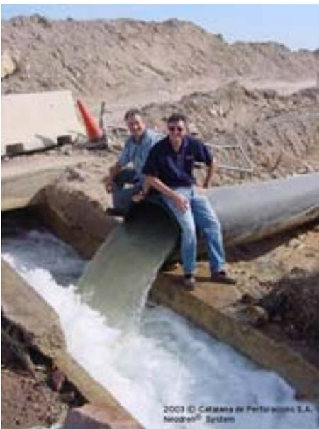
Figure 6: Example of seawater supply through Neodren® system.
