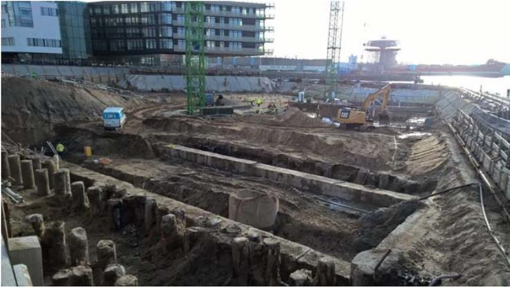
Figure 2: slurry walls of the subway tunnel crossing the building site
