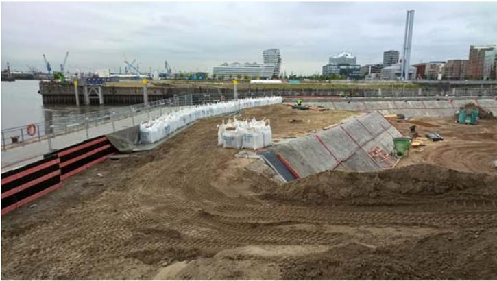
Figure 6: construction of the protection against storm floods
