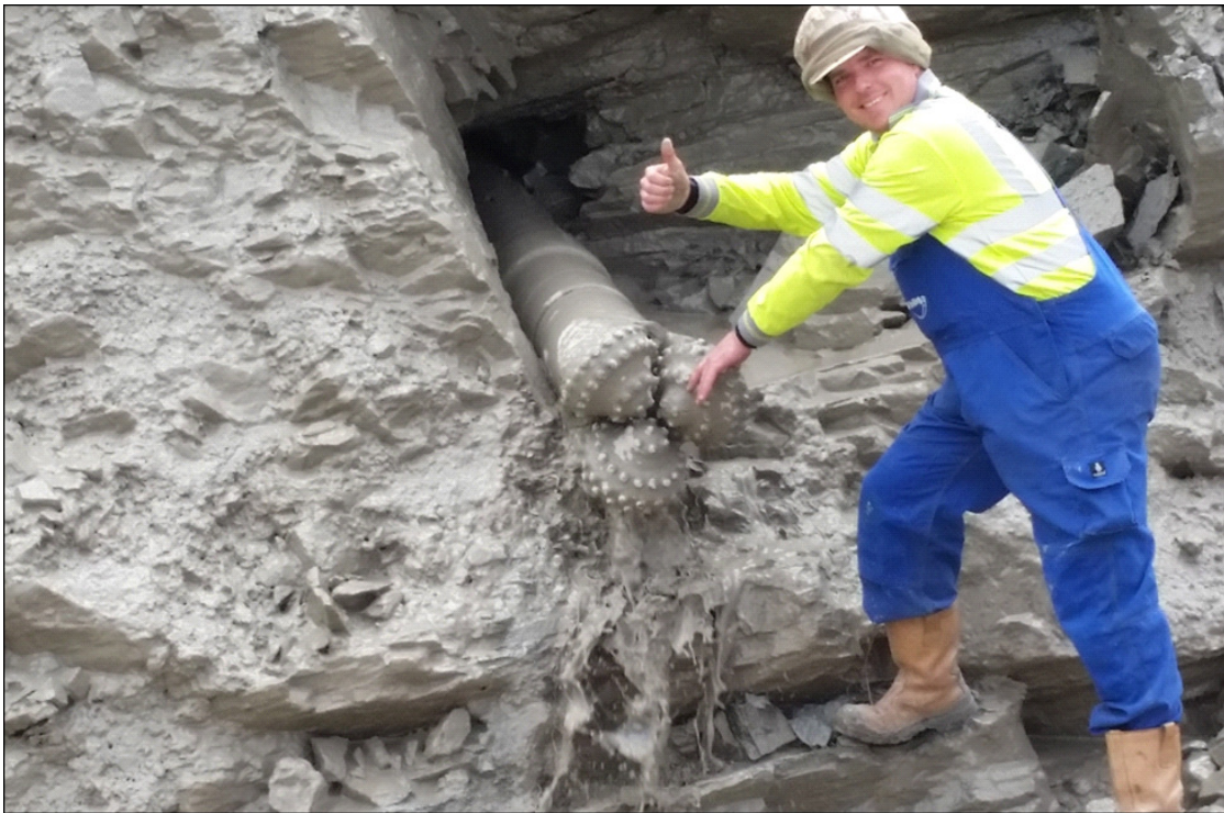
Fig. 3 Completion of Pilot Drill
