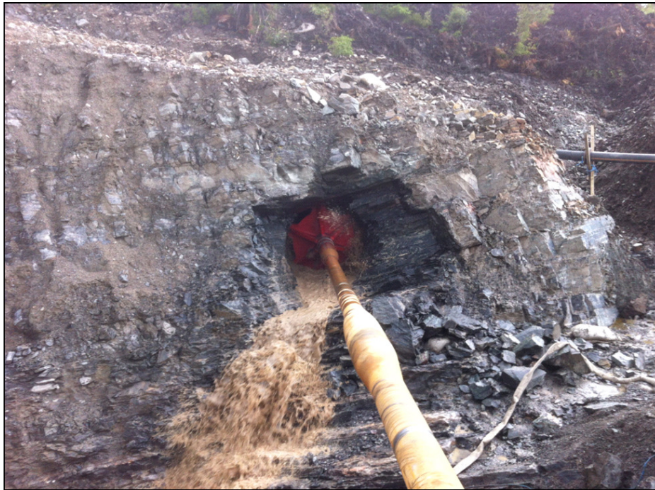
Fig. 4 Start of 38" Hole-Opening Pass
