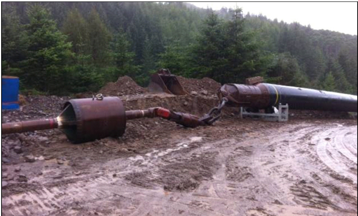
Fig. 7 Ready for Pullback
