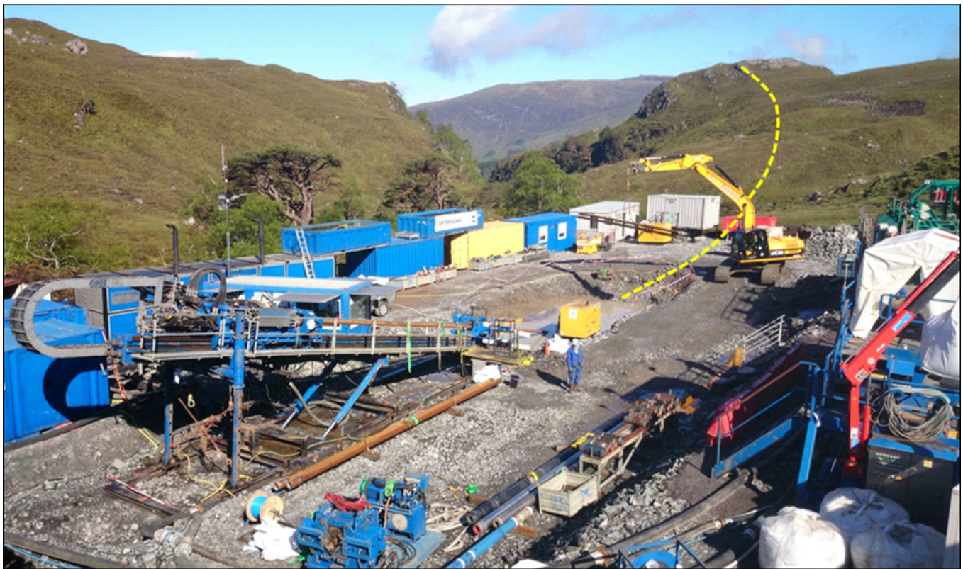
Fig. 2 HDD Drill Site showing Drill Alignment
